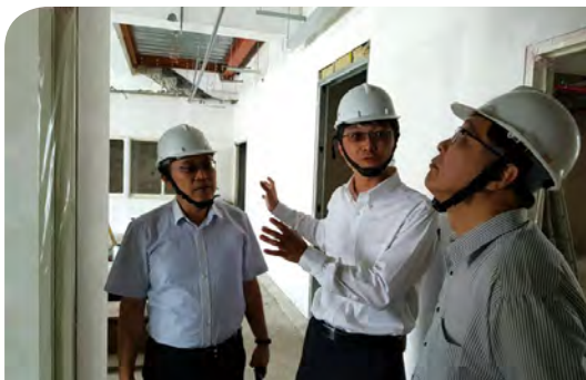
■ Director-General Cheng, Ming-Chian inspected the Liuhe Barrack Office Building construction site
