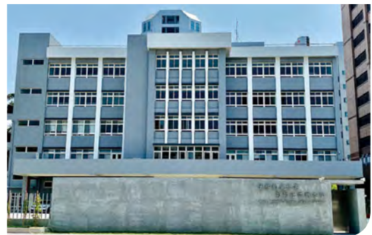
■ Liuhe Barrack Office Building of Southern Investigation Office, Construction Completed
