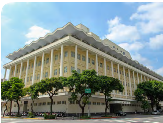
■ AAC Headquarters (including the Northern Investigation Office) in Bo'ai Building
